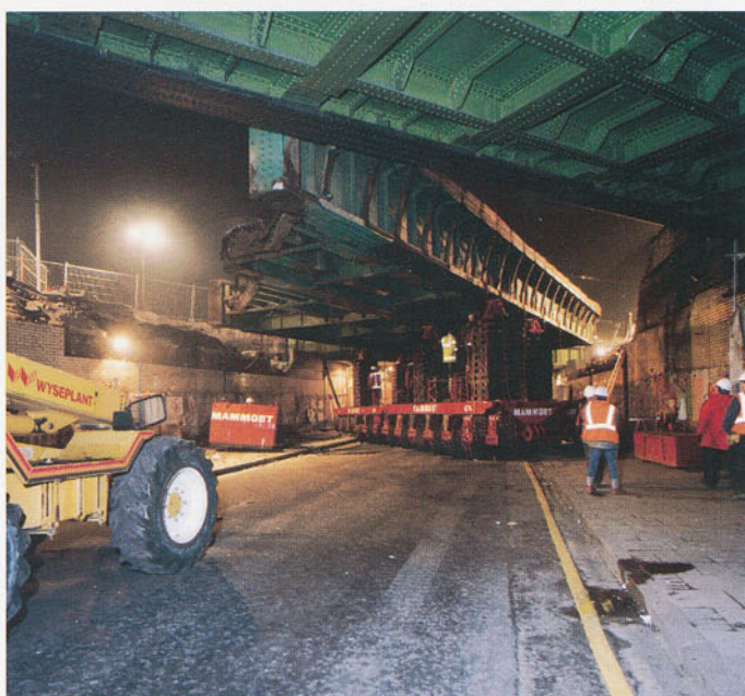
London — Mammoet Transport (UK) Ltd exchanged an old bridge section for a new one at Finsbury Park in two consecutive night shifts. The picture shows the old bridge being carouselled from its foundations by self-propelled modular transporters. Afterwards it would be jacked down and driven off the site.
