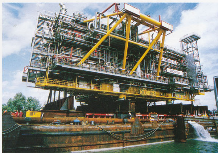
Zwijndrecht — Mammoet's electronic weighing system certified the weight of the Harald West A Topsides facilities module, built at Grootint in Zwijndrecht. Exactly 4,787 tonnes were rolled out of the workshop on SPMTs and moved onto an ocean-going barge.
